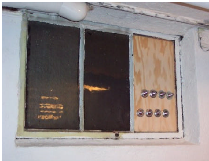
Basement Window With Inside Bulkhead Panel
